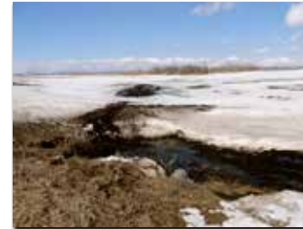
Culverts cleaned out early spring.
