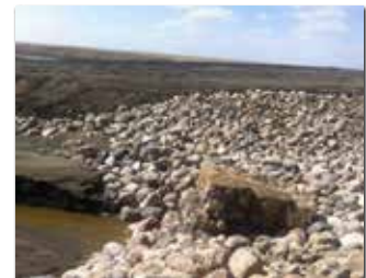
More rock added at an erosion control drop structure.
