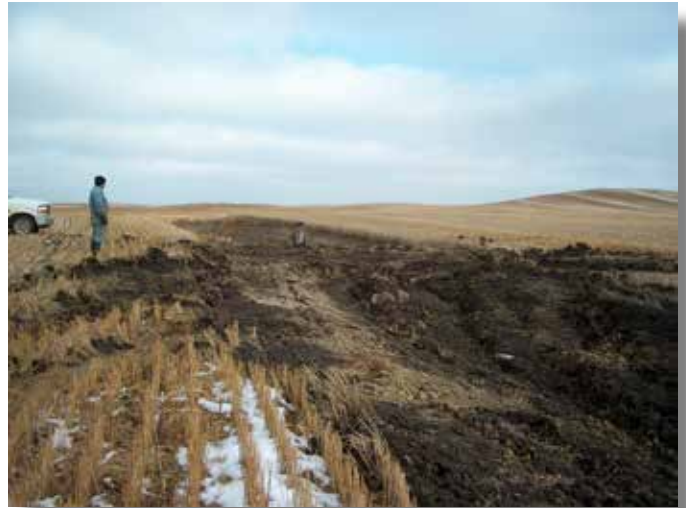
Figure 2. This photo is an example of a drainage works that was closed in response to a RFA by installing a ditch block. Respondent is now in compliance with The Water Security Agency Act .
